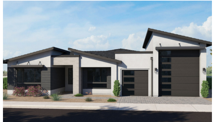
Contemporary Elevation with Opt RV Garage
